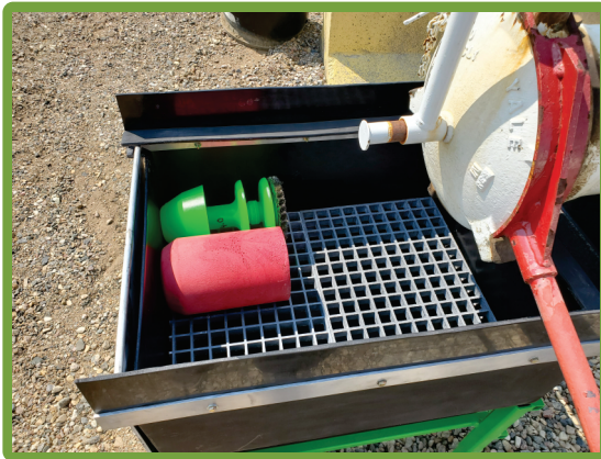
Wind guards to prevent liquids from being blown and spilt on the ground
